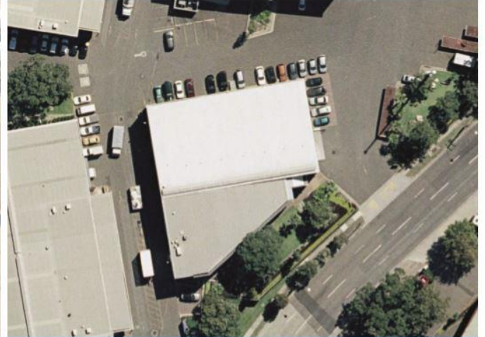
When SkyCool was applied to the warehouse roof of Cosmax Prestige Brands, internal temperatures fell significantly.
